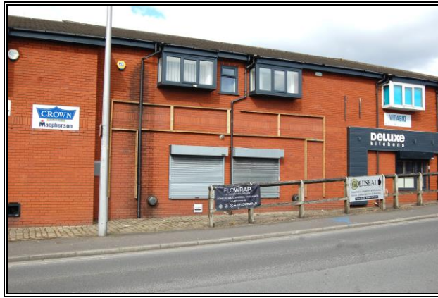
Frontage to George Street
